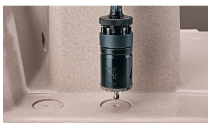
B - Align the drill with pre-punched hole
